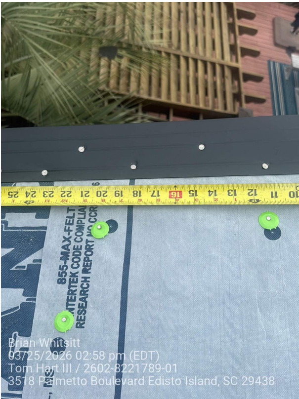
Photo Documentation: Documentation of the nailing of the Drip Edge.
