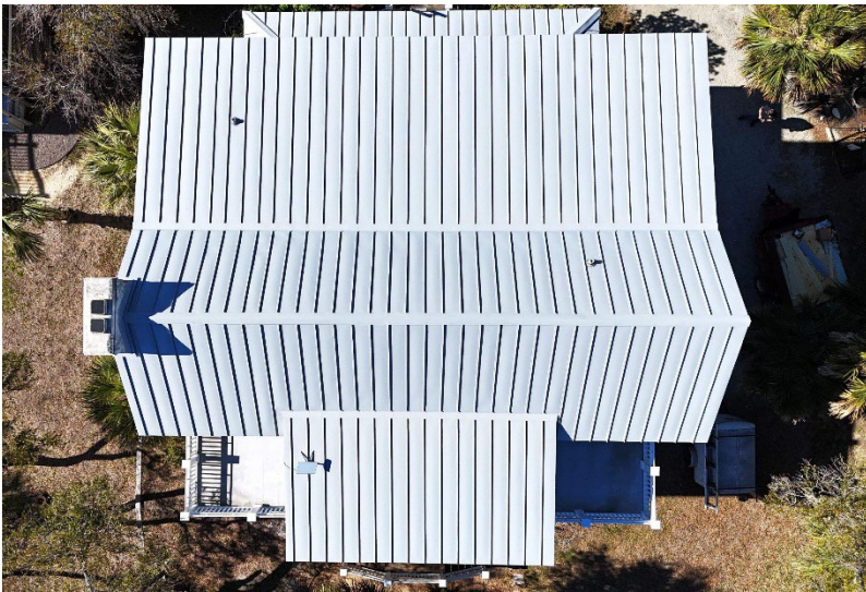
Photo Documentation: Drone Photo of completed metal roof installation
