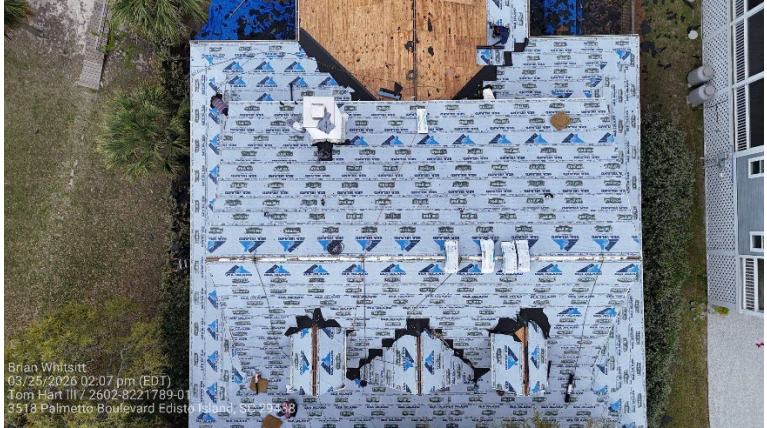
Photo Documentation: Drone photo showing secondary water barrier installation
